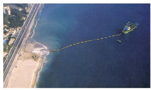
Figure 3. One soft solution is the replenishment of sand, won from a marine bank, by a hopper dredger.
